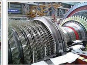
Blade Ring Assembly & Clearance Check
